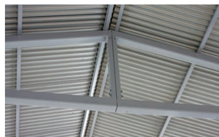
Weather protection against sun and rain.
